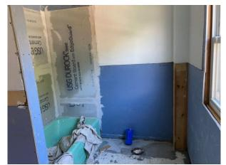
The last big project is the upstairs bathroom. All of the old, green tile has been removed, new concrete board and purple board has been put up, and the walls and floors have been prepped for tile. And we're started to lay the tile.
